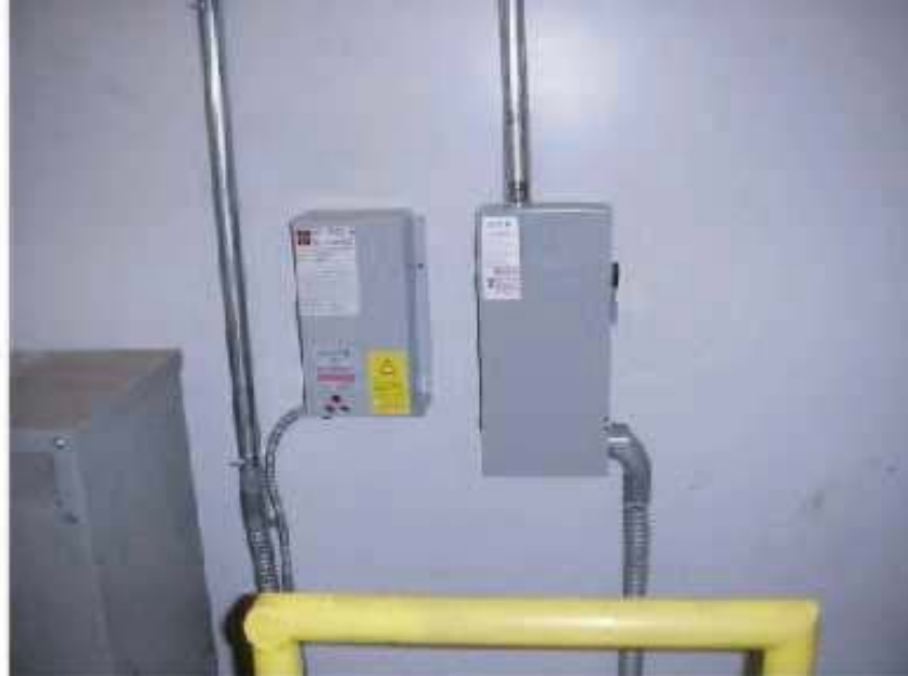
7.5 KVAR Located at the load
