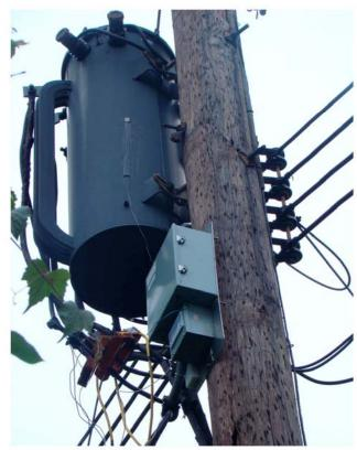
Pole Monitors at Hilltop Terrace. Monitor 10 services one building at Hilltop Terrace and a second building in a different complex. Monitor 11 services five buildings at Hilltop Terrace. The transformer at Monitor 10 is a 75 KVA, 3 phase transformer. The transformer at Monitor 11 is a 150 KVA, 3 phase transformer. Both transformers date to the construction of the complex in 1965.
